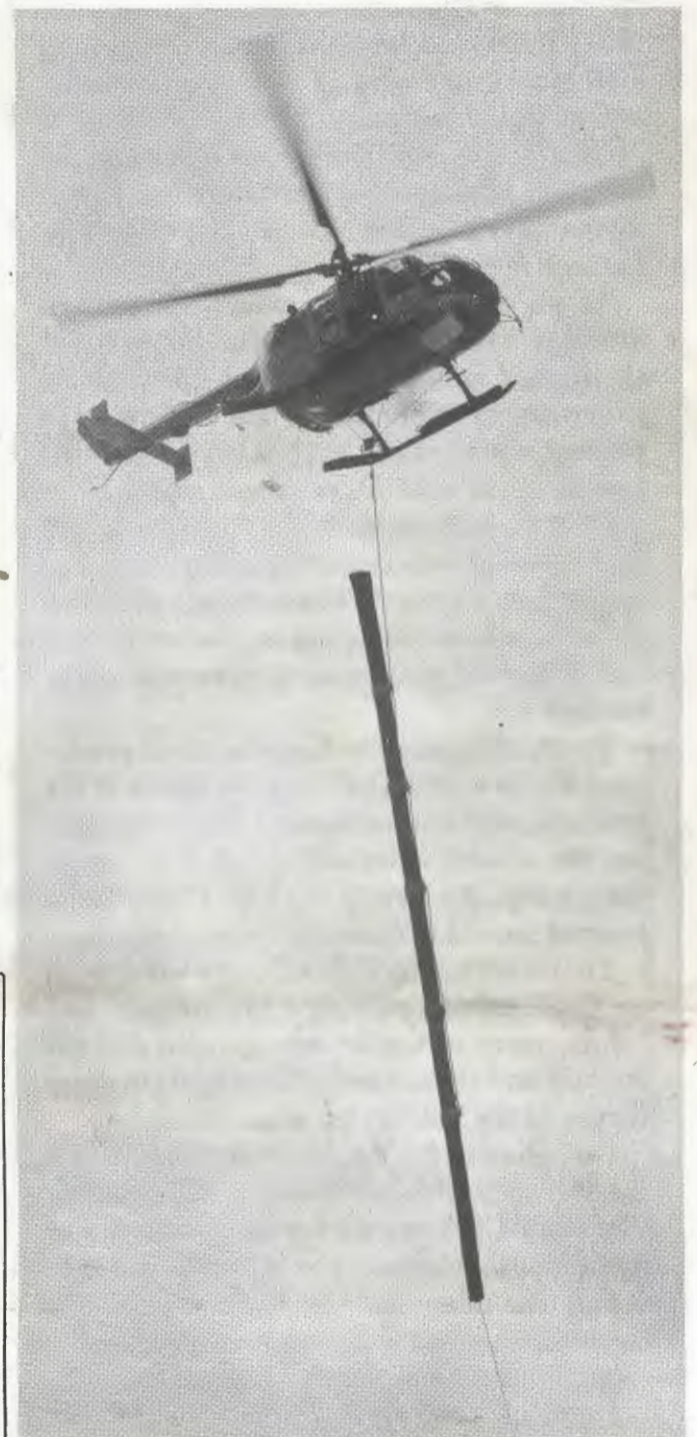
Air Lift to South Stack
