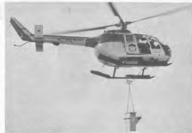
The Trinity House helicopter carries the transformer to its site.
